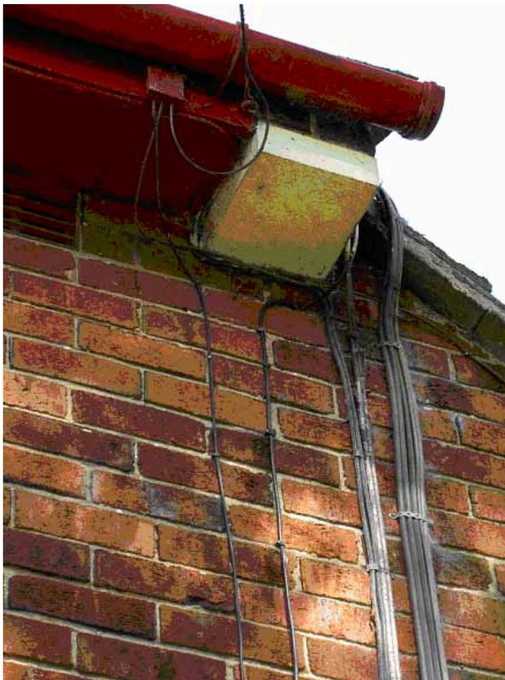
Later, a more detailed conversation with the homeowners revealed the cables to be the domestic supply cables for the property. They ran the full length of the front of the house at eaves level before dropping down to the wall to enter the meter / distribution box. A further set of cables continued to supply the farm outbuildings and milking parlour.
